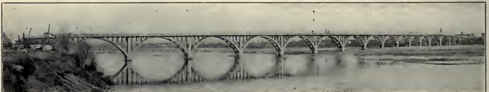
THE NEW REINFORCED CONCRETE ARCH BRIDGE AT FORT SMITH, ARK.
